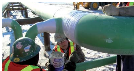
Application of Protal 7125, low temperature pipeline coating.
