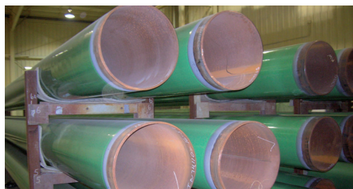
Jet fuel pipelengths stockpiled prior to installation at the airport.
