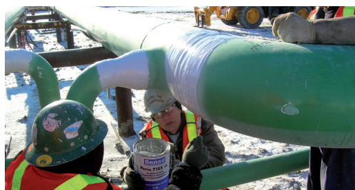
Application of Protal™ 7125, low temperature pipeline coating.
