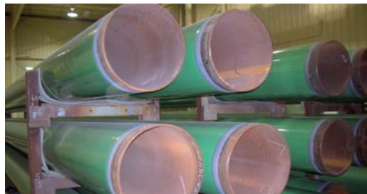
Jet fuel pipelengths stockpiled prior to installation at the airport.
