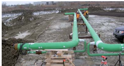
With no preheating necessary, the girth welds can easily be coated with Protal 7125 at temperatures of -15°C.
