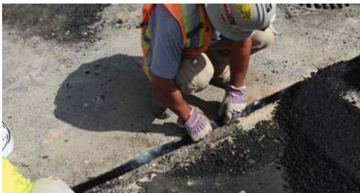
Densoband is applied to the vertical joint face of the reinstatement trench providing a waterproof and flexible seal over the entire depth of the joint.
