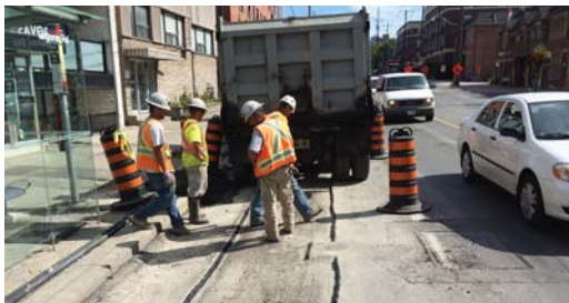
The Densoband in place along both of the vertical joint faces of the reinstatement trench.
