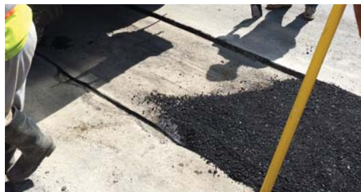
Application of the new asphalt road surface.
