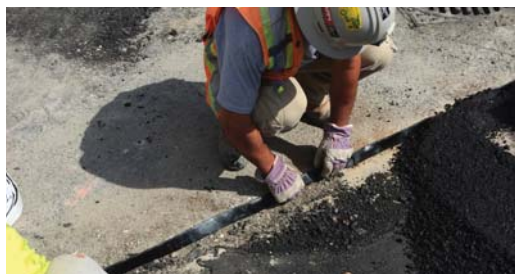
Densoband is applied to the vertical joint face of the reinstatement trench providing a waterproof and flexible seal over the entire depth of the joint.
