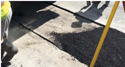
Application of the new asphalt road surface.
