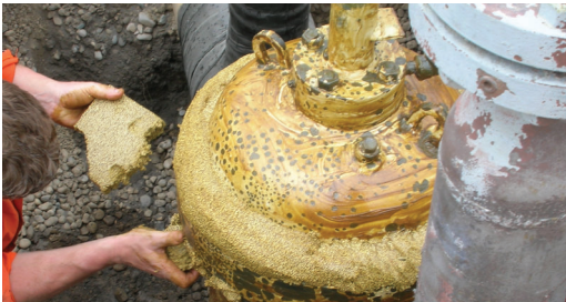
Denso Profiling Mastic is used to fill voids and smooth all irregular contours ready for wrapping with Denso LT Petrolatum Tape.
