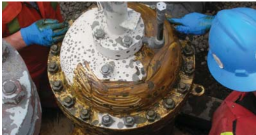
Denso Paste used to prime surface to displace moisture and penetrate rust before applying mastic and tape.
