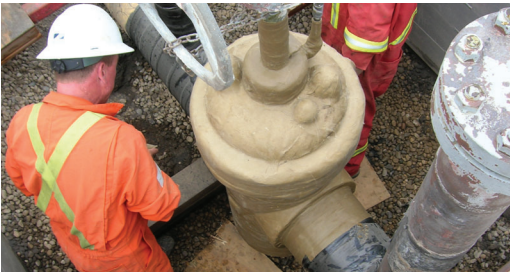
A final wrap of Denso LT Petrolatum tape to finish the job - note the flexibility of the tape and ease of wrapping over awkward shapes.
