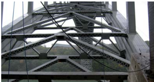
Denso Void Filler protecting straddled cable supports from corrosion
