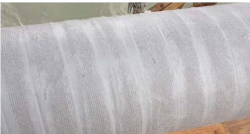
Denso ColorTape was used as corrosion prevention measure as well as a lead encapsulation means.
