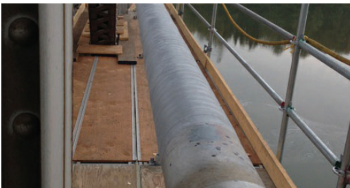
DensoColor Tape is easy to install and requires no special training to apply.
