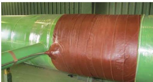
55% overlap of Denso Hotline Tape around the sensor to provide corrosion protection prior to being buried.
