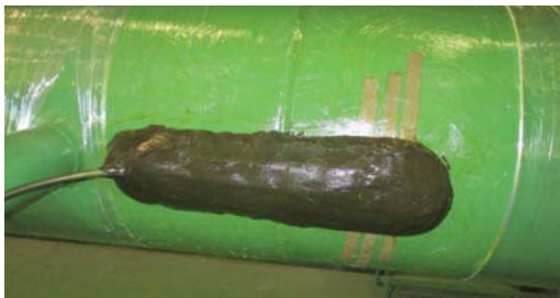
The RTD Sensor is encapsulated within Densyl Mastic.
