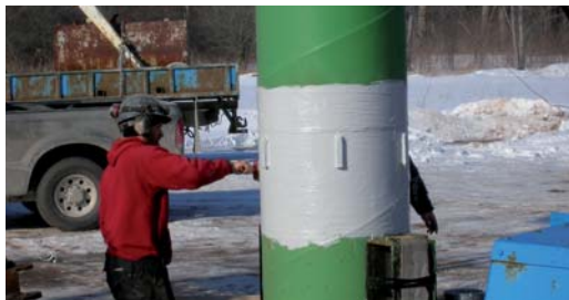
Girth weld area being coated with Protal 7125 in sub-zero temperatures.
