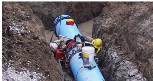
Valves being prepped prior to the Denso Petrolatum Tape System applied.
