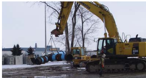
Water pipelines, with Denso LT Tape, being transferred.
