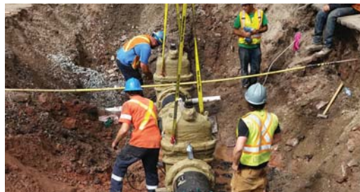
New water valves being protected by Denso LT Tape.
