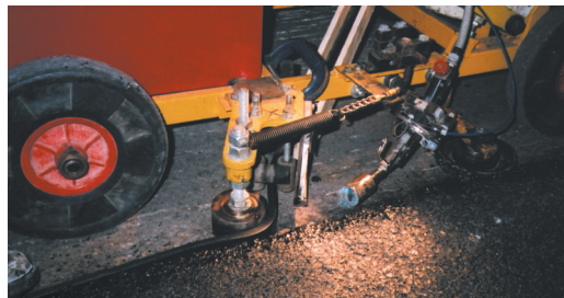
Close up of the Densoband™ applicator machine.
