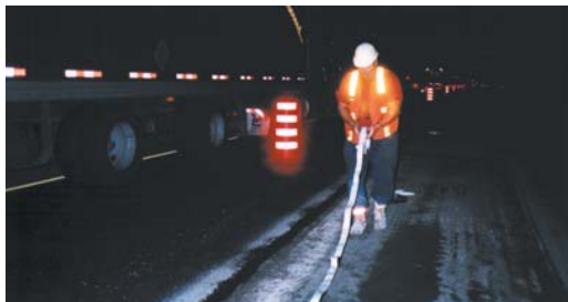
Densoband comes in several sizes. 15mm x 45mm x 6.5m rolls were used on this project.
