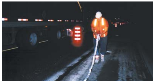
Densoband comes in several sizes. 15mm x 45mm x 6.5m rolls were used on this project.
