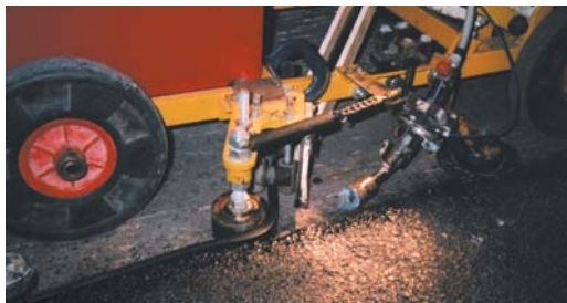
Close up of the Densoband applicator machine.
