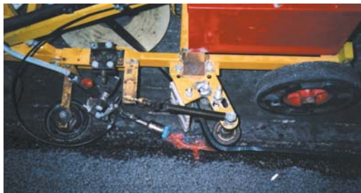
Applying Densoband at 360metres/hour with the special Densoband applicator machine.
