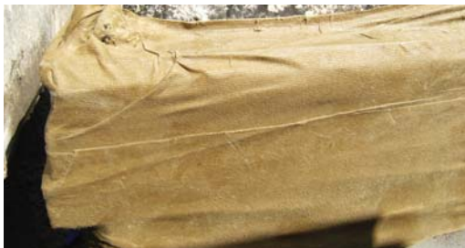
Denso Petrolatum Tape preventing water ingress and road corrosion around municipal castings.
