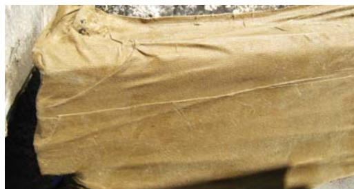
Denso Petrolatum Tape is loaded with material so will remain water proof even when concrete below cracks.
