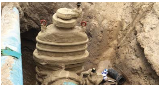
The valve is wrapped with Denso Petrolatum Tape to complete the protection.
