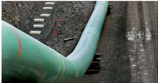
The pipelengths are welded together and the welded joint areas are then coated with Denso Protal 7200 before being buried.
