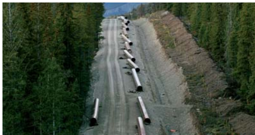
Pipe lengths awaiting Denso Protal application, mark out the route through the stunningly beautiful and environmentally sensitive Canadian National Park.
