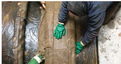
The Denso Petrolatum Tape System will adhere to metal, concrete, PVC and polyethylene substrates.
