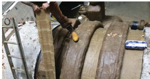
Denso LT Tape is easily spiral wrapped by hand over large diameter fittings.
