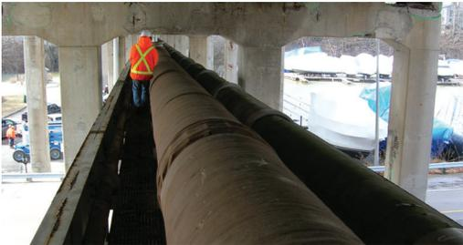
75ft. above a local parking lot the tapes were supplied and the underside applied by an operator on a lift truck.
