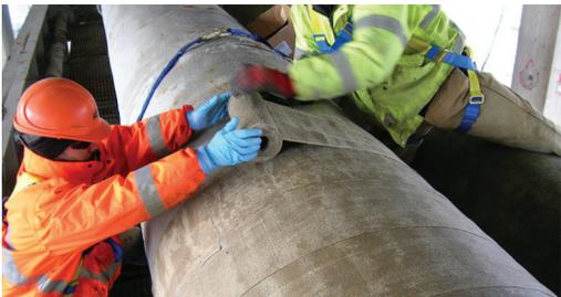
Denso LT Tape was applied in a short amount of time to concrete pipe, providing reliable protection.
