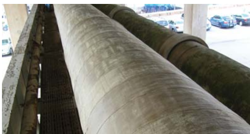
The concrete pipeline wrapped with Denso LT Tape.
