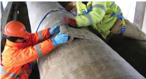
Denso LT Tape was applied in a short amount of time to concrete pipe, providing reliable protection.
