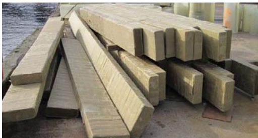
Rectangular timber headers were wrapped with Denso Petrolatum Tape.
