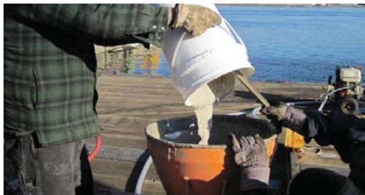
SeaShield 550 Epoxy Grout being loaded into the peristaltic pump.
