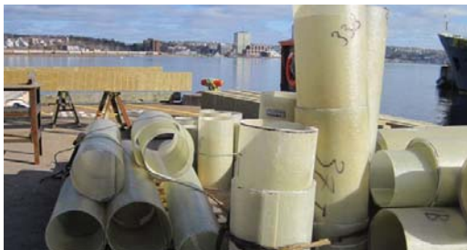
SeaShield 500 FRP jackets ready for installation.
