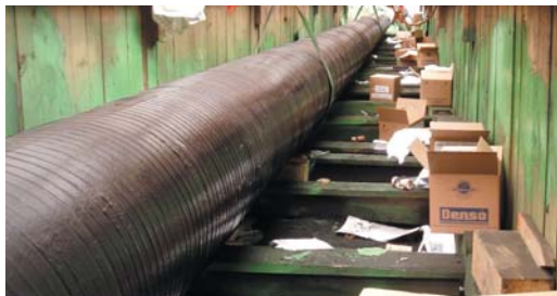
30" gas line protected with Protal 7250 overwrapped with Densopol Tape
