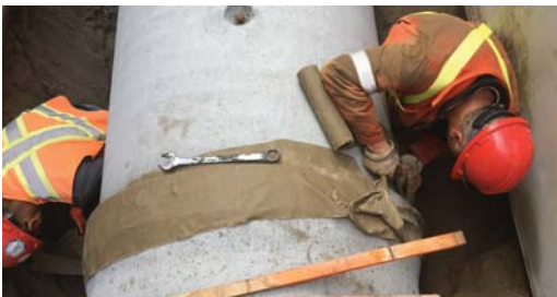
Workers sealing the Denso LT Tape by hand, ensuring that all air is pushed out and seams are closed, providing a water tight seal.
