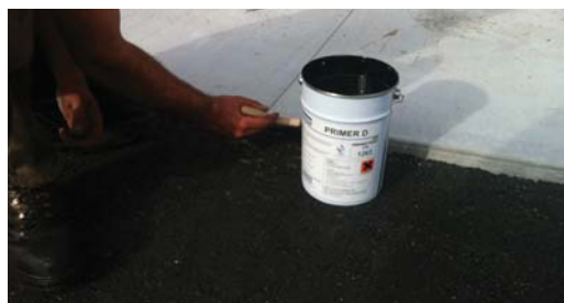
Denso Primer D, a bitumen primer, is applied to the concrete prior to installing the DensoBand along the joint.
