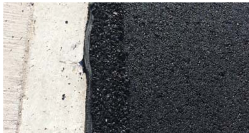
DensoBand provides a uniform, watertight, flexible seal.
