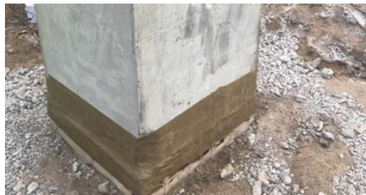
Hi-Tack Tape is applied 6" below to 6" above the joint and will provide a permanent flexible water-tight seal.
