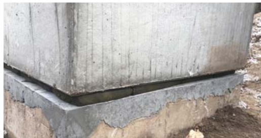
Densyl Mastic is laid upon the prepared surface in preparation for the box chamber.
