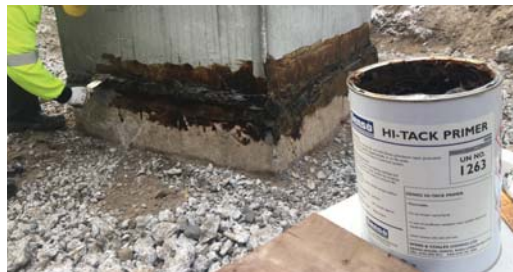
With the chamber in place, Hi-Tack Primer is applied in thin uniform coating.
