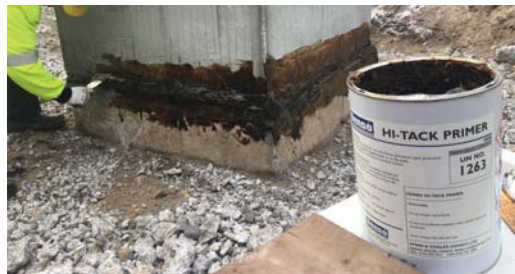
With the chamber in place, Hi-Tack Primer is applied in thin uniform coating.
