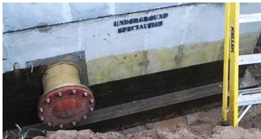
Denso Hi-Tack Paste and Tape is applied from the bottom up.
