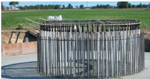
Rebar rods being installed on site.
