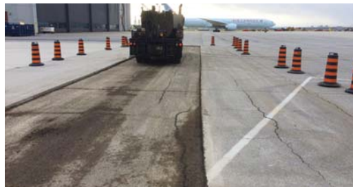
Section of taxiway being prepped for repairs.
