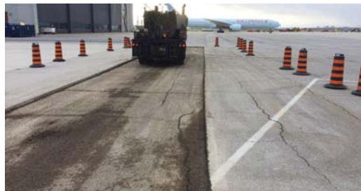
Section of taxiway being prepped for repairs.
