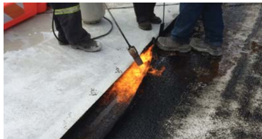
DensoBand is used for sealing hot asphalt to cold joints including asphalt, concrete and steel.
