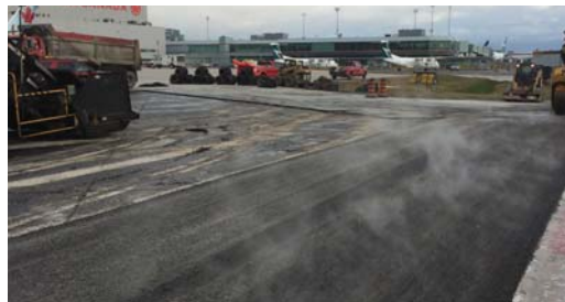
Repaired patch where the DensoBand will withstand future asphalt movement and thermal expansion.
