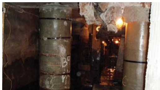
Completed Denso Fiber-Forms installation to the timber piles.
