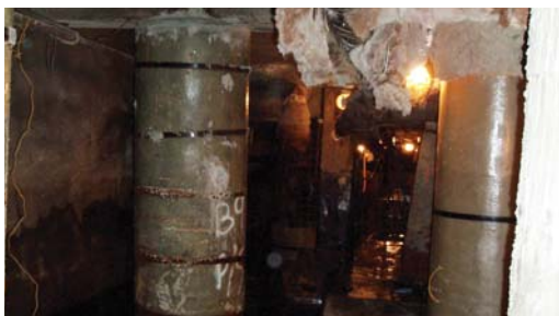
Completed Denso Fiber-Forms installation to the timber piles.
