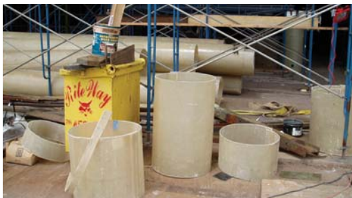
Uninstalled SeaShield Fiber-Forms being prepped and awaiting install.
