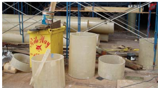
Uninstalled SeaShield Fiber-Forms being prepped and awaiting install.
