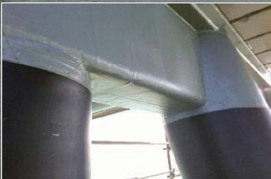
The Denso Steelcoat 400 System was used to protect the headstocks.
