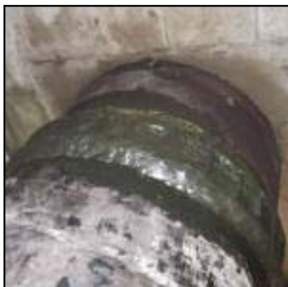
Application of Denso Mastic.
