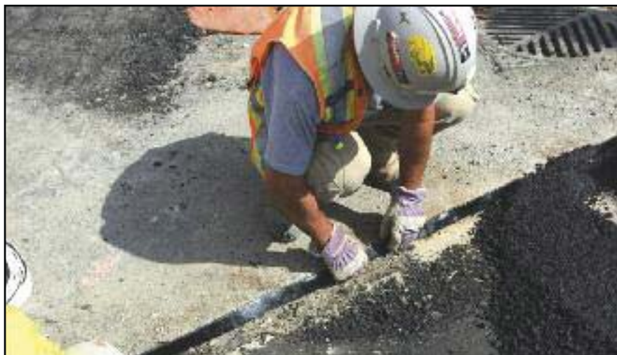
Densoband is applied to the vertical joint face of the reinstatement trench providing a waterproof and flexible seal over the entire depth of the joint.
