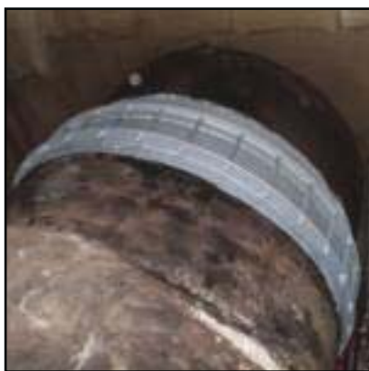
Application of paint primer.
