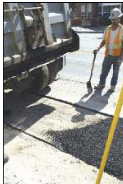
Application of the new asphalt road surface.
